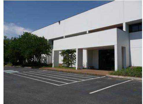
The exterior surface is comprised of textured tile-up concrete panels with stained accents. Horizontal reveals and vertical fin walls were incorporated to provide solar shading and define the office entrance.
