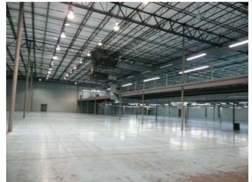
Office area was approximately doubled within the existing building mezzanine, and structural elements in the warehouse, including mezzanine floors and exterior walls, were modified to coordinate with new distribution equipment.
