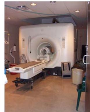
An existing MRI room and associated control area was enlarged and reconfigured to accommodate a new, more powerful scanner. Existing walls, floor slabs, and ceilings were re-worked with new lead shielding as required for the greater magnetic fields.
