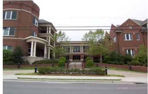
The 46,000 square foot expansion is comprised of a three story, post-tensioned concrete structure with sub-surface parking. The residential quality of the neighborhood required a traditional approach to the architecture of the exterior facade.
